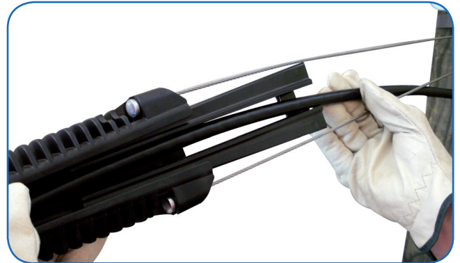
The clamp body is placed over the cable with the wedges in their back position
